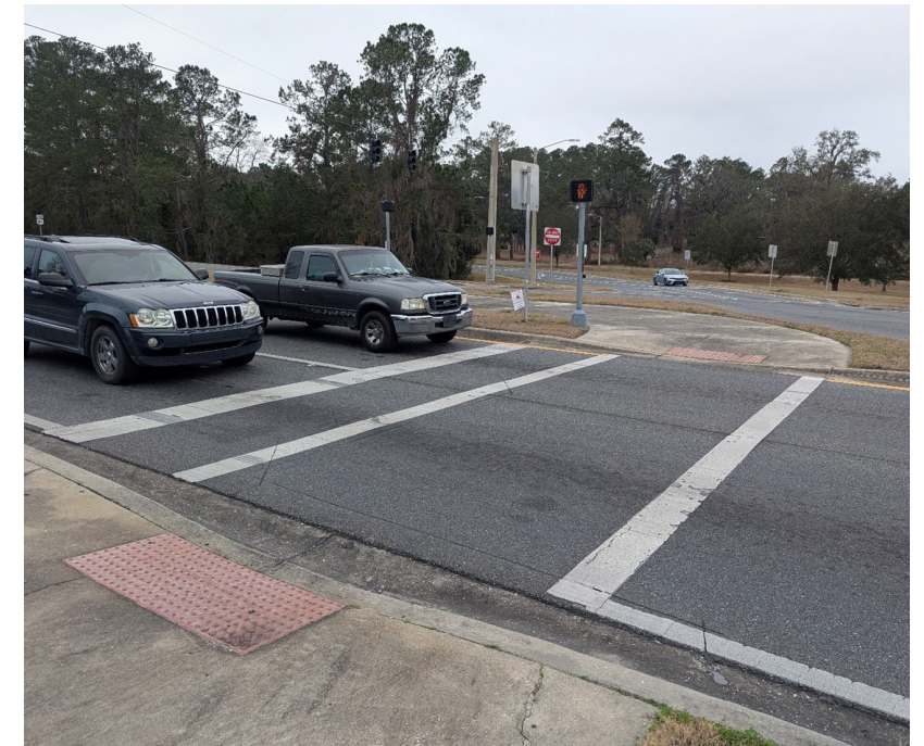
SHORT DISTANCE FROM NORTHBOUND STOP BAR TO CROSSWALK
