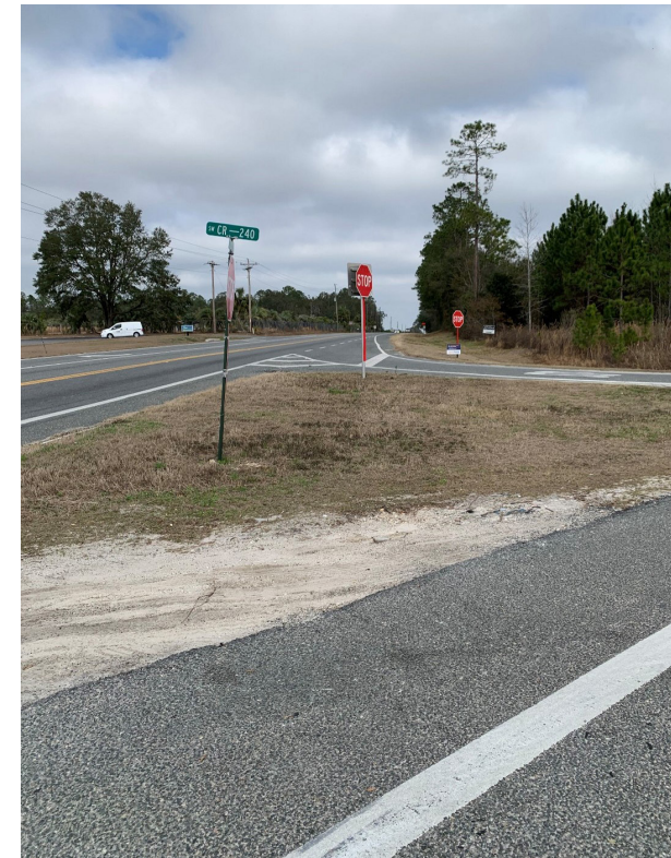
HILL TO THE NORTH OBSTRUCTS VIEW OF VEHICLES TRAVELING WESTBOUND, WESTBOUND RIGHT VEHICLES FURTHER BLOCKS VIEW OF SOUTHBOUND VEHICLES
