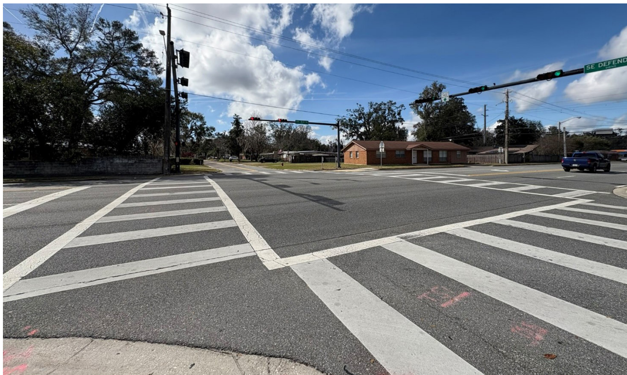
SIGNALS AT SE BAYA DRIVE & SE DEFENDER DRIVE (LACK RETROREFLECTIVE SIGNAL BACKPLATES)
