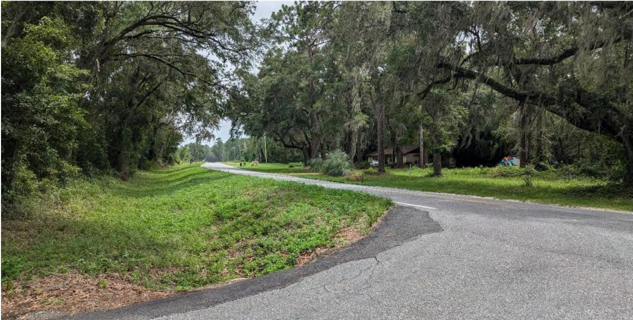
Sight distance from SE Leslie Wood Ln WB stop bar facing South
