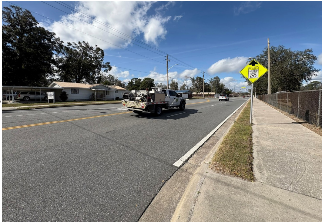
SR 10A (SE BAYA DRIVE), FACING WEST
