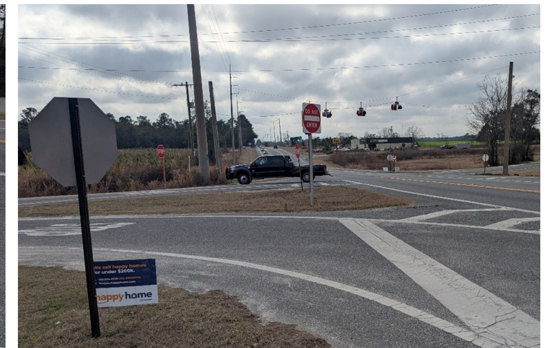
CAN ADD AN ADDITIONAL DO NOT ENTER SIGN ON THE BACK OF THE STOP SIGN
