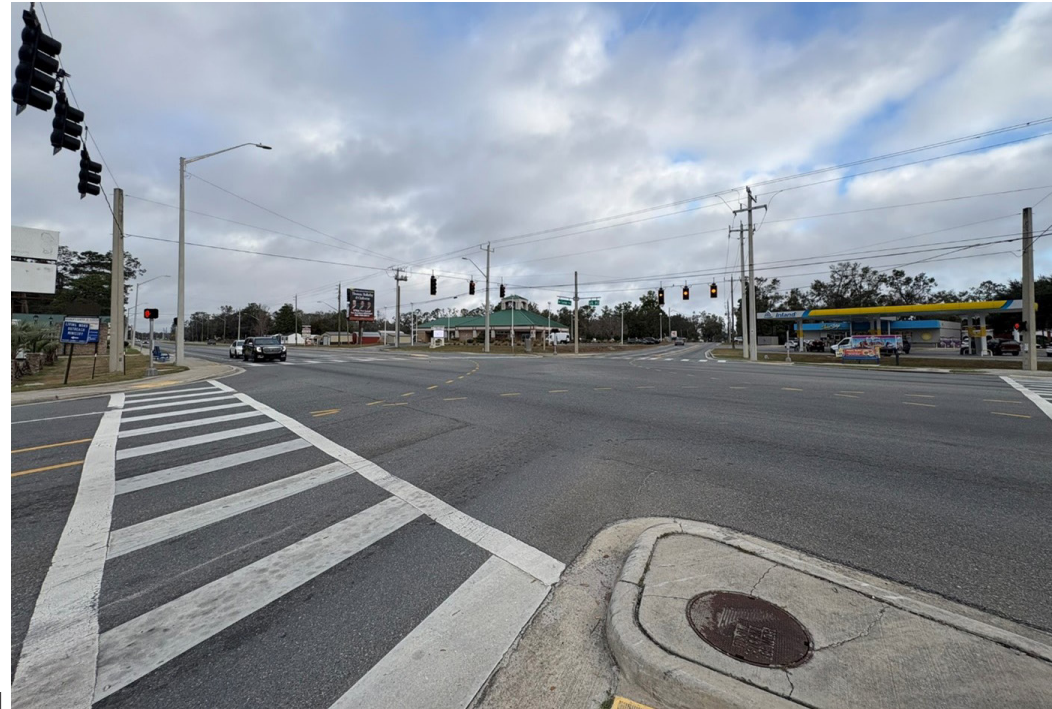
INTERSECTION OF US-90 & SW PINEMOUNT ROAD/NW TURNER AVENUE (VIEW FROM SOUTHEASTERN CORNER)
