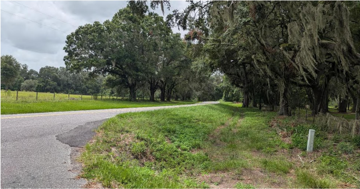
Sight distance from SE Leslie Wood Ln WB stop bar facing North
