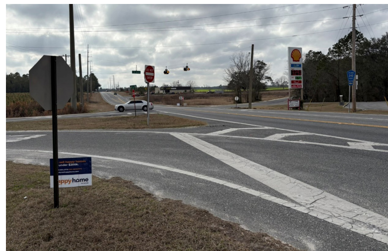
SOUTHBOUND LEFT MOVEMENT IS DANGEROUS DUE TO LACK OF TURN LANE AND DOWNGRADE SLOPE
