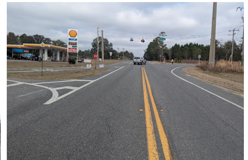
VIEW OF NORTHBOUND APPROACH
