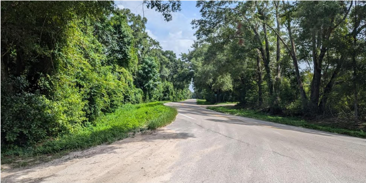
Sight distance from SW Truluck Terrace WB stop bar facing West
