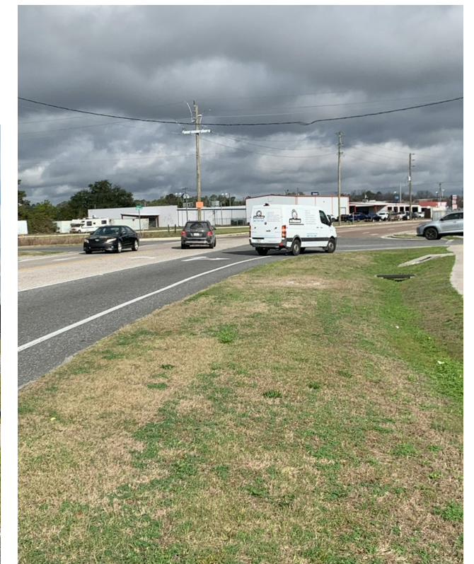
TURNS FROM MAJOR APPROACHES TIGHT FOR TRUCKS
