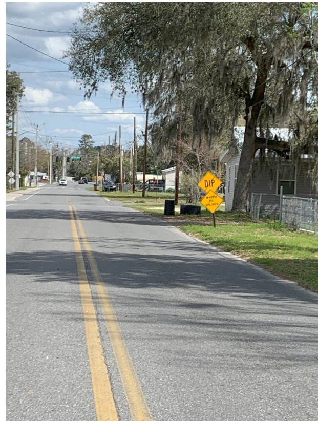
NO DELINEATION BEFORE ROADWAY ENDS ON SOUTHSIDE OF ROAD
