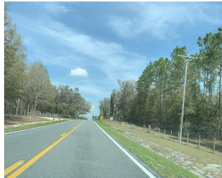
LACK OF LIGHTING ALONG SW TUSTENUGGEE AVENUE
