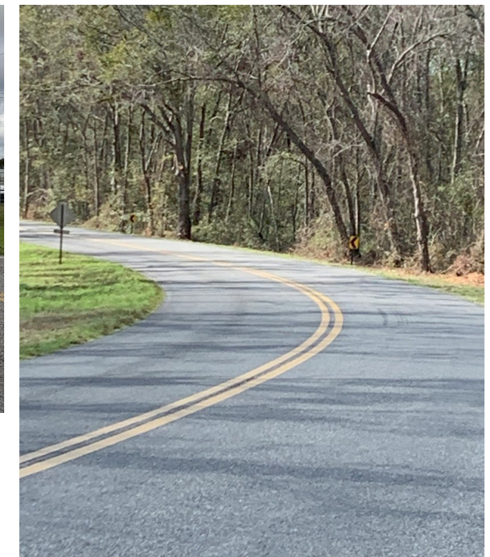
CHEVRON SIGNS ON NORTHERN CURVE
