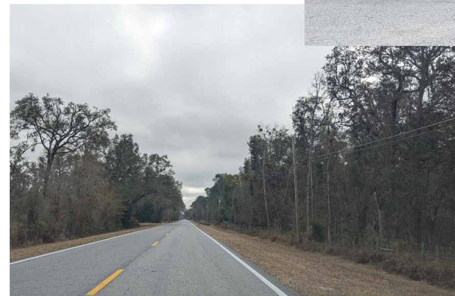
UTILITY LINES FOR POTENTIAL LIGHTING IMPROVEMENTS
