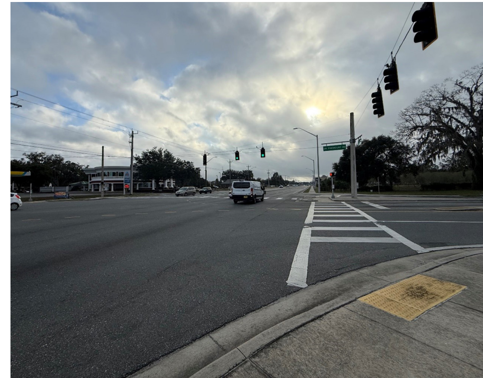
PEDESTRIAN SIGNALS AT CHANNELIZING ISLAND (DOES NOT COVER THE ENTIRE PEDESTRIAN CROSSING)
