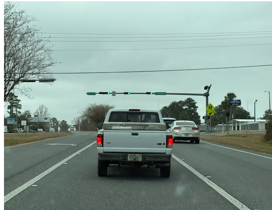
PEDESTRIAN SCHOOL SIGN WITH LIMITED VISIBILITY AND LIGHTING
