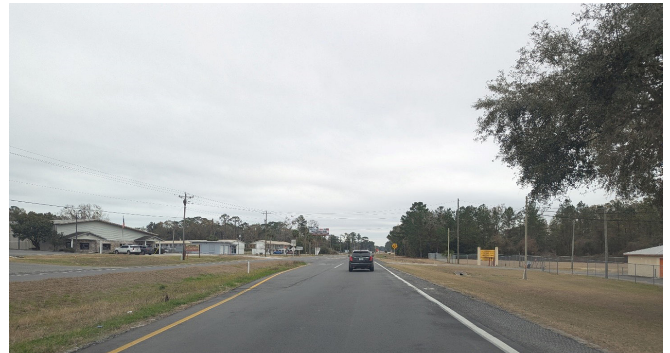
LACK OF LIGHTING
