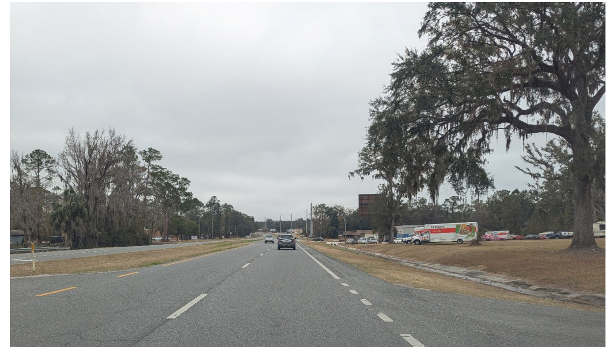
LACK OF LIGHTING
