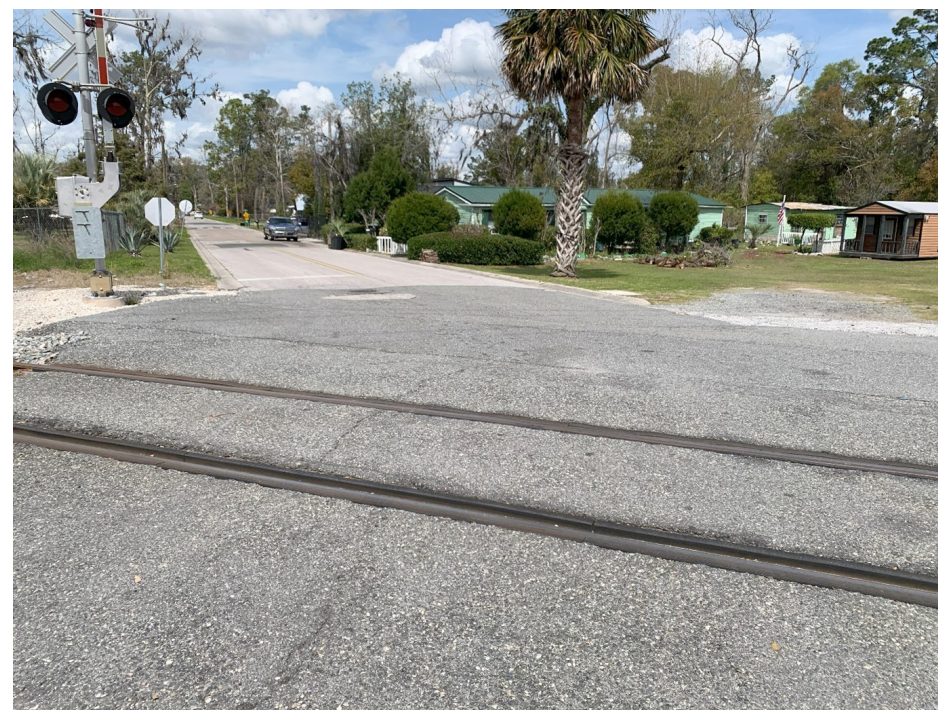
SOUTHBOUND STOP BAR AT RAILROAD CROSSING
