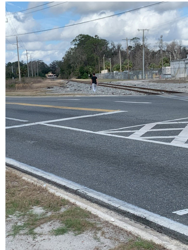
PEDESTRIAN NEAR TRAIN TRACKS WITHOUT PROPER FACILITIES
