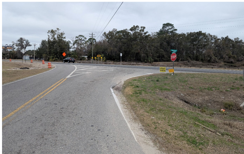
VIEW OF APPROACH TO INTERSECTION OF SW FOREST LAWN WAY WITH US 41
