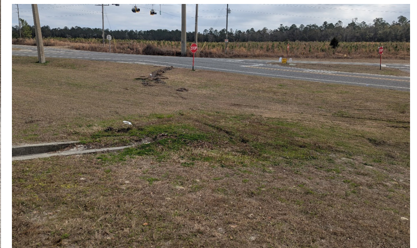
POTENTIAL OFF-ROAD TIRE MARKS
