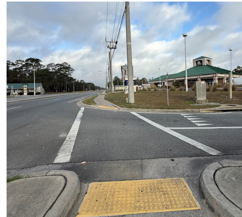
MISSING PEDESTRIAN MARKINGS ON NORTHERN LEG
