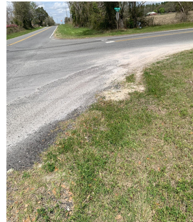
RIGHT-TURN RUTTING FOR NORTHBOUND RIGHT-TURN MOVEMENT AT SW TUSTENUGGEE AVENUE AND SW CR 240
