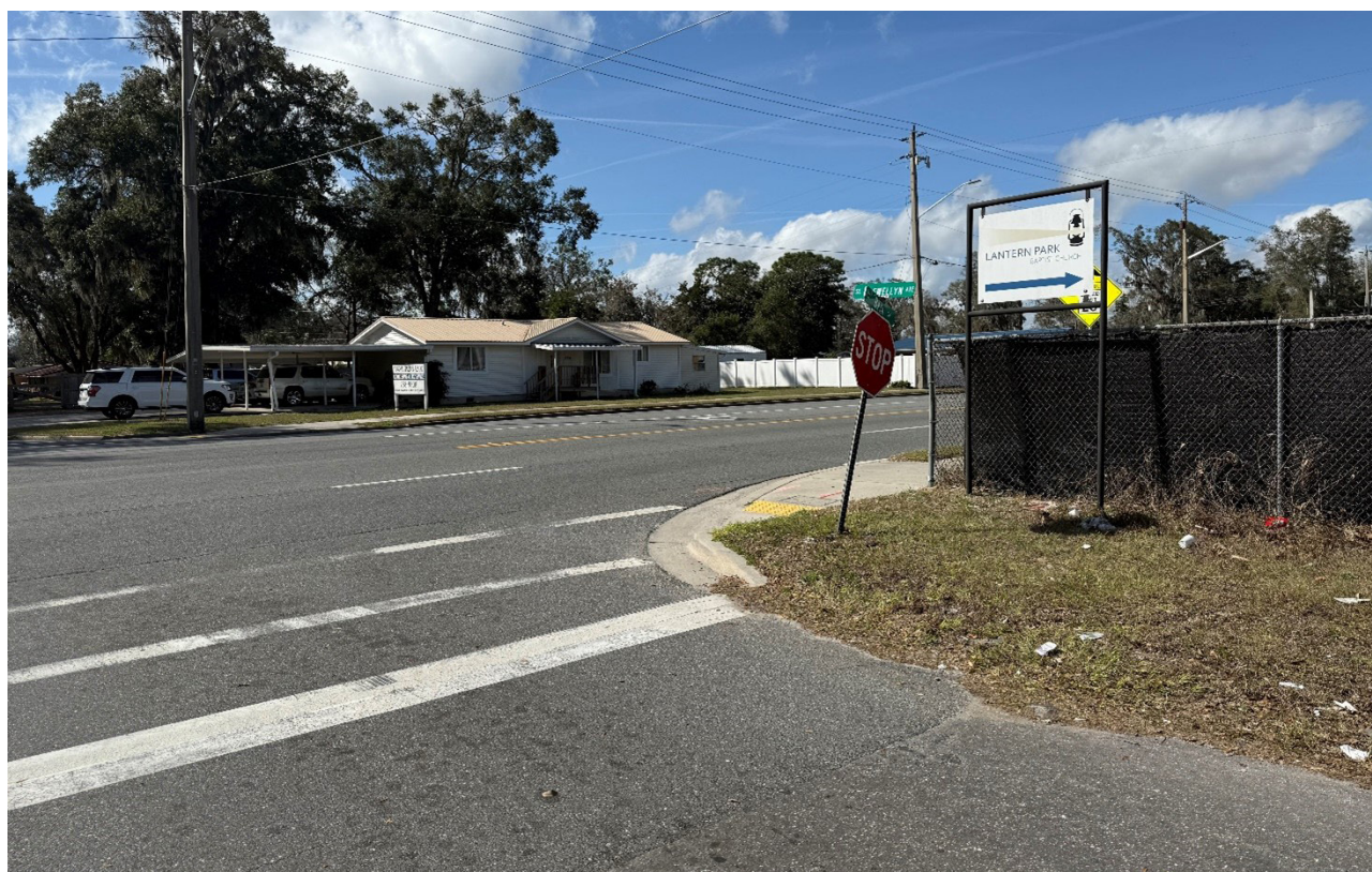
FENCE BLOCKS VIEW ON SOUTHBOUND APPROACH FOR SE LLEWELLYN AVENUE
