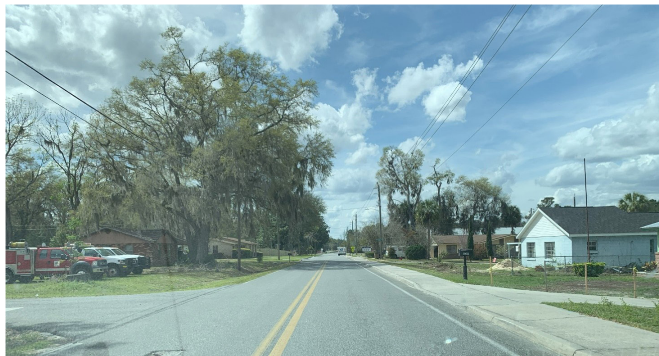
CURB IS INCONSISTENT ALONG ROADWAY
