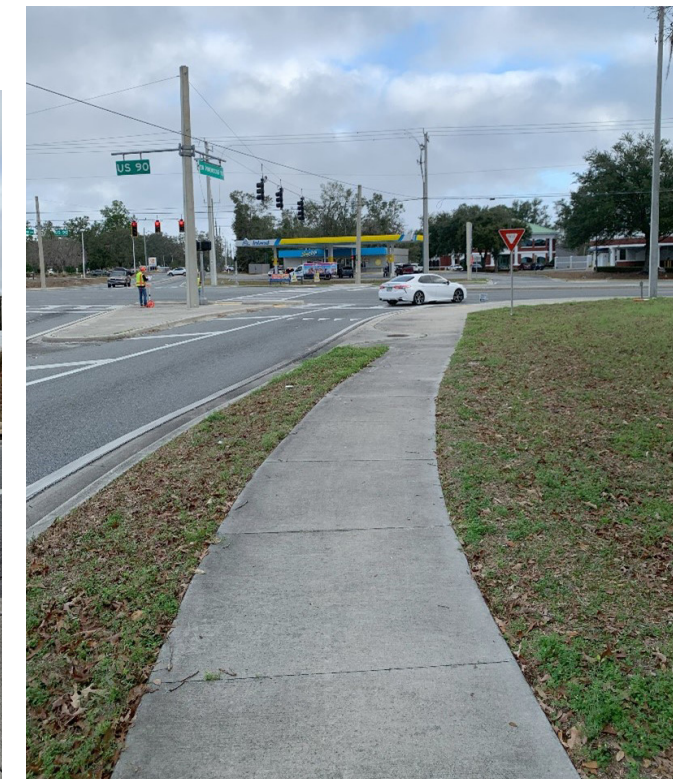
VIEW OF CHANNELIZED RIGHT TURN ISLAND
