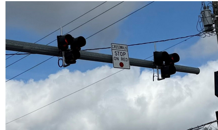
SIGN ON HAWK CROSSING NEEDS CLARIFICATION FOR BLINKING RED SIGNAL
